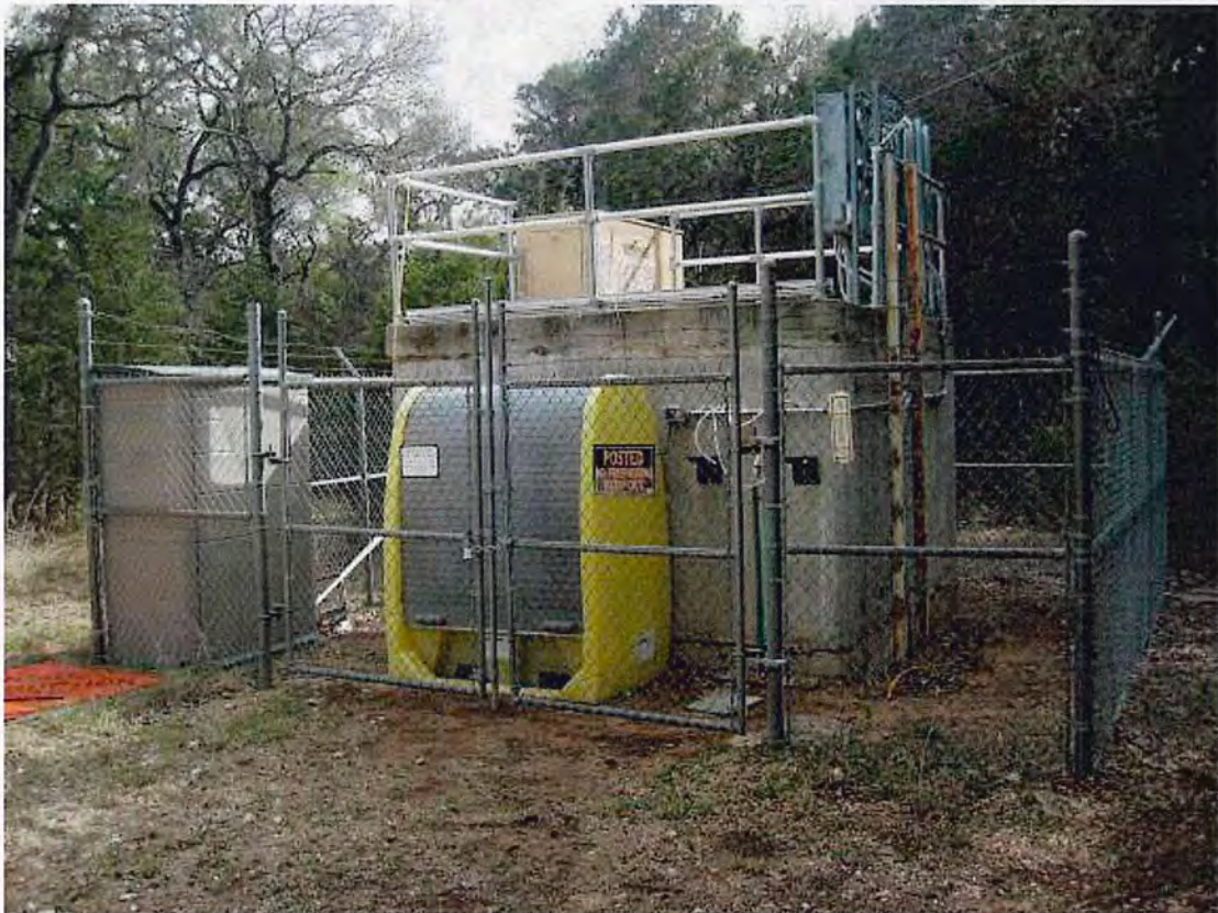
Photo 2. Existing wastewater treatment plant lift station
