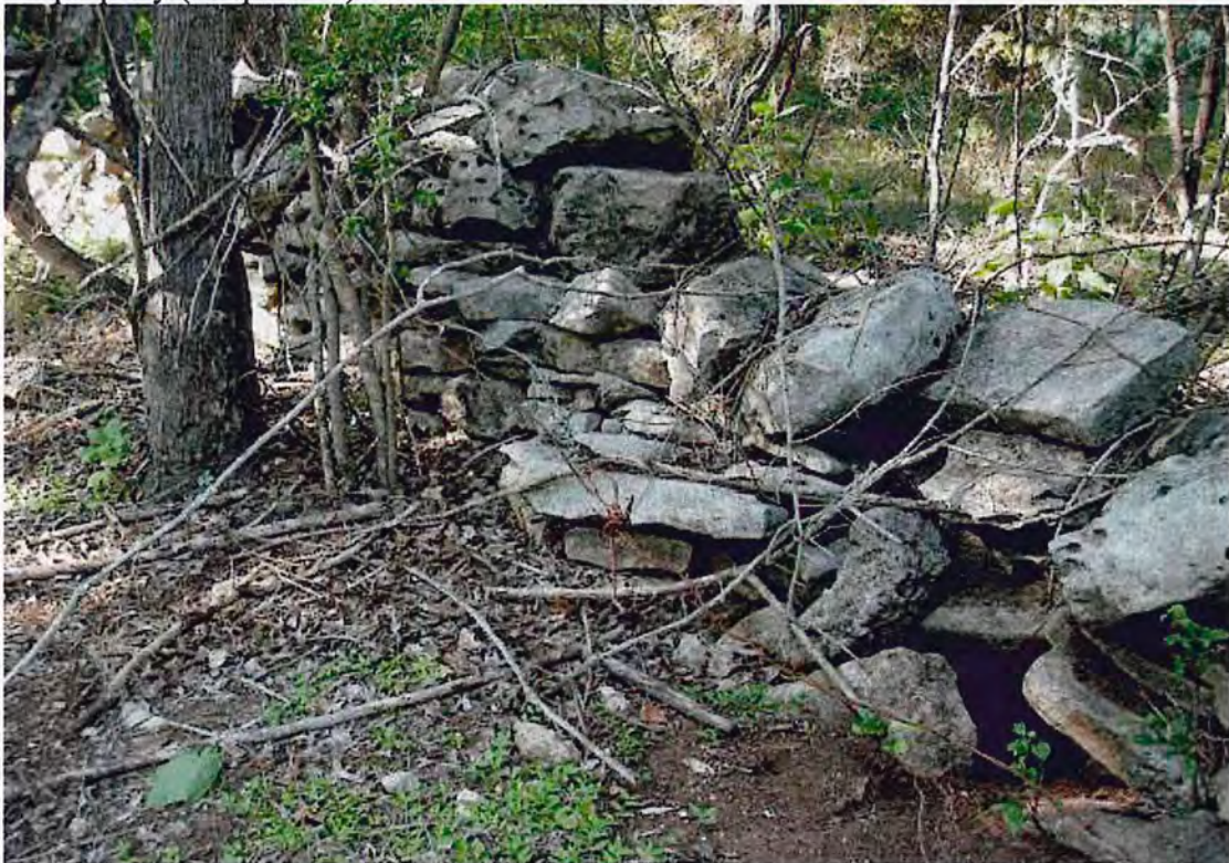
Photo 3. Existing dry-stack rock walls
